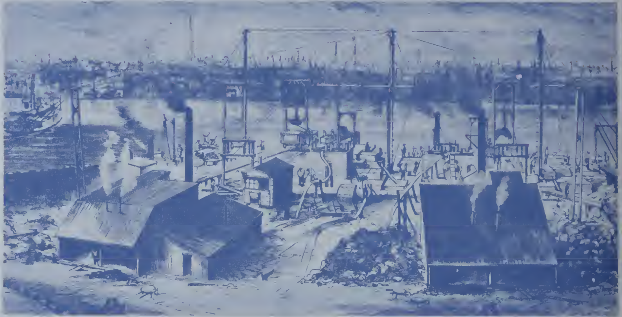
The Brooklyn pier begins to take shape, the first courses of stone being placed on top of the timber caisson.
